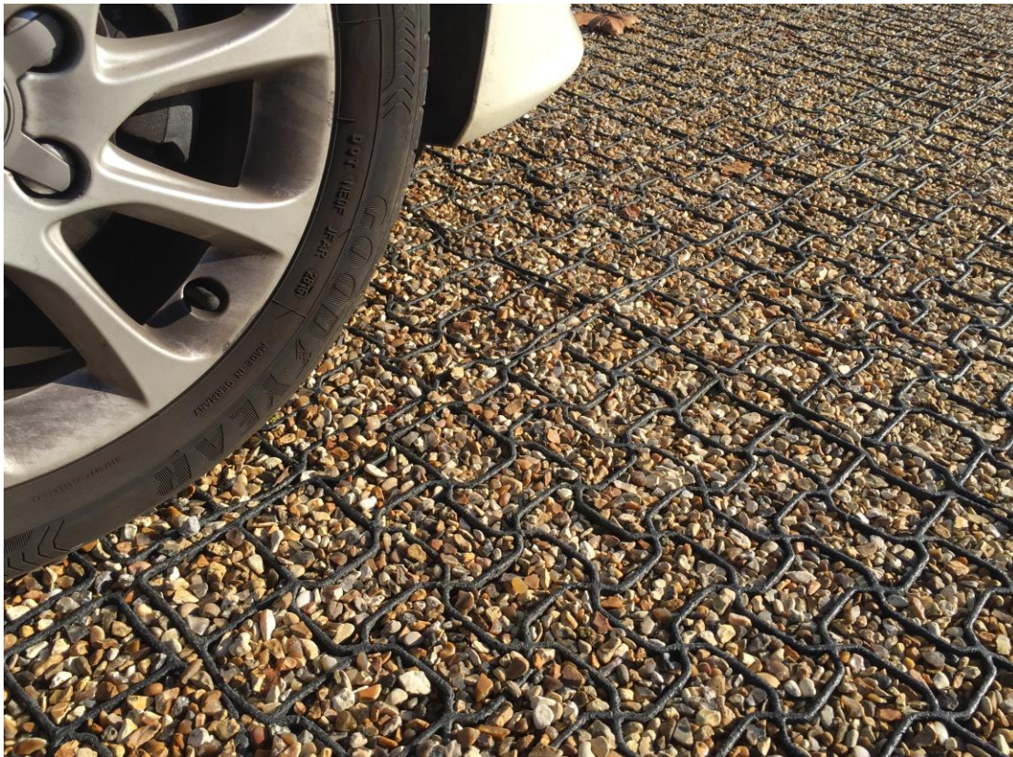
Photo 4: An example of a finished Gravel Grid system
