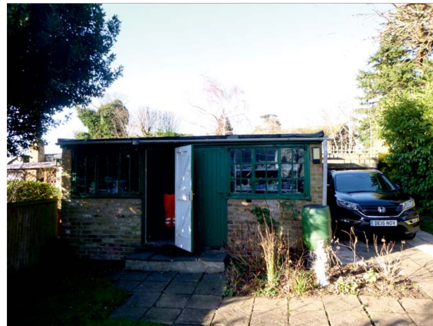
Photograph 4: Showing the garage.
